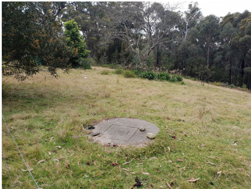
Photo 4 Looking east towards the eastern side of the site, near BH02, note inground septic tank and grade of slope in an easterly direction (Photo taken 29 August 2022).
